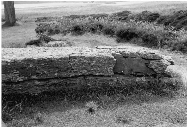
Fig. 9. This is a photograph of a sandstone monument that toppled when it was struck by lightning in 1980. Spalling is observed at its base, at the right of the photograph; and the deep midwidth fracture extends the full 4 m length of this stone. A partial view of one of the remaining 27 upright stones in this historic Ring of Brodgar, located in the Orkney Islands, UK, is observed in the upper left corner of the photograph.
